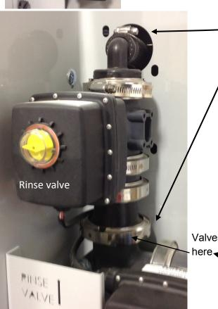
Remove these two clamps to remove the rinse valve assembly. The rinse valve assembly will go inside the cabinet after valves 5 & 6 are attached.
