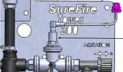
Pressure Sensor (3 wire type) with harness 521-05-050150
